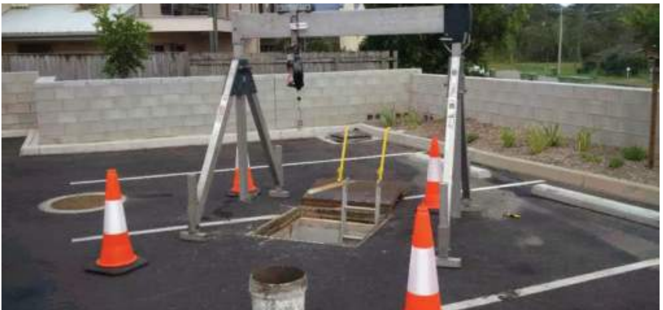
FIGURE 4 SPELFilter install set-up
